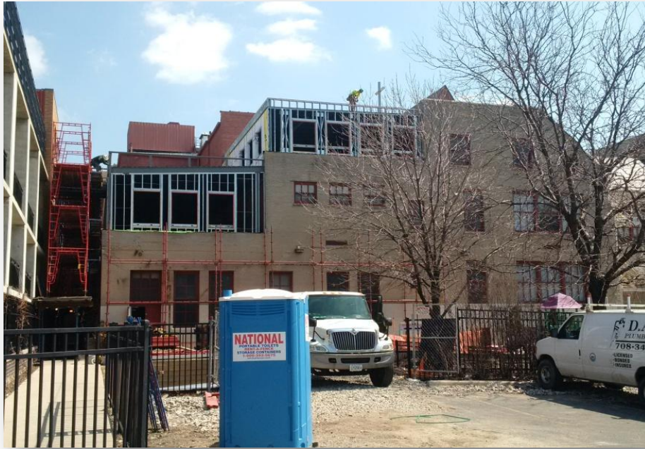
Classroom additions in progress
