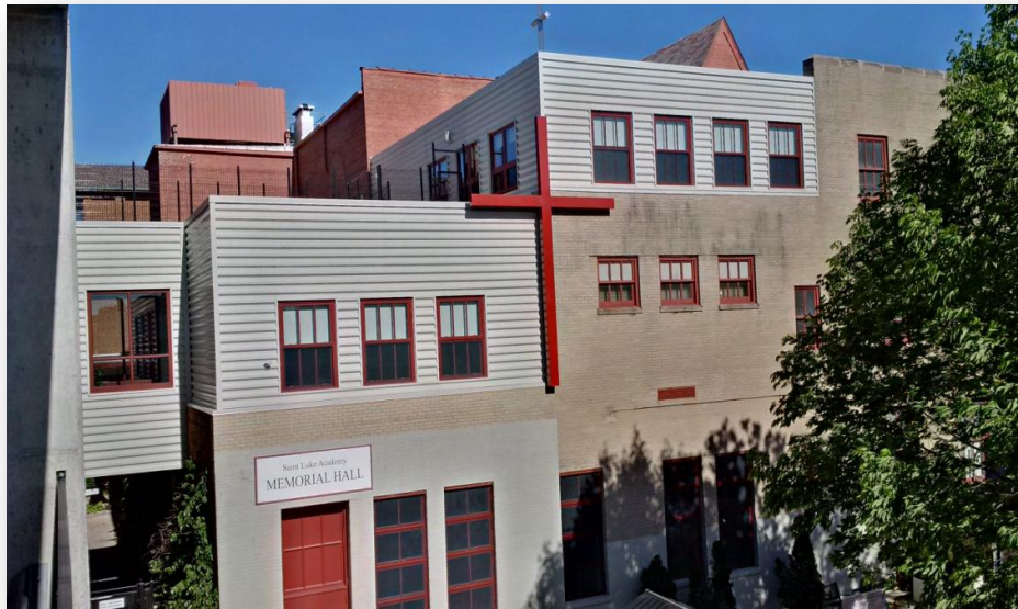
Classroom additions & bridge to the garage / elevator lobby after the additions were completed
